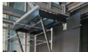
③ Shielding door installation
