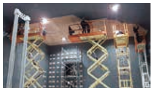
⑦ Ferrite tile construction
