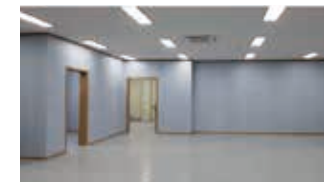
⑫ Internal, external interior finishing
