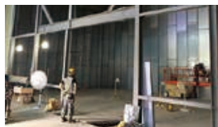
② H-Beam and shielding panel construction
