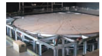
⑥ Turn table construction
