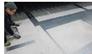
⑩ Internal interior construction
