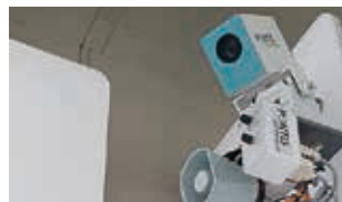
⑨ CCTV installation
