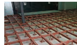
⑤ Raised Floor construction
