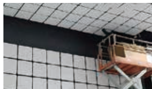
⑧ Hybrid absorber construction
